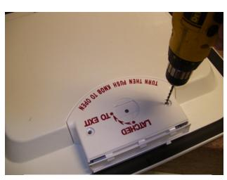
STEP 4. Using a 5/32" drill bit, carefully drill through the center of the plastic rivet. Remove both rivets.
